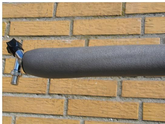
**Note:** Always ensure the earth-connection is present in the socket outlet and connected to the heating cable. Also ensure the installation is connected to an RCD max. 30mA. If the plug and socket outlet is not matching, change the plug or use an adaptor, to ensure the product is fully earthed.
