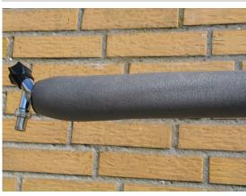
**Note:** Always ensure the earth-connection is present in the socket outlet and connected to the heating cable. Also ensure the installation is connected to an RCD max. 30mA. If the plug and socket outlet is not matching, change the plug or use an adaptor, to ensure the product is fully earthed.
