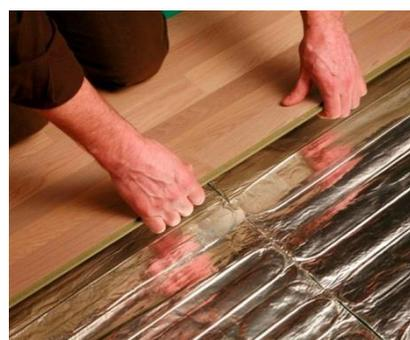
Fig. 11) Laying the wooden floor
