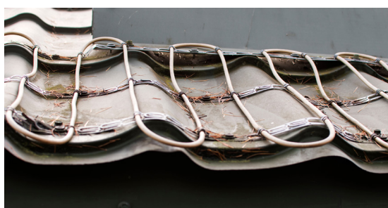
34000003 - screwed onto roof surface
