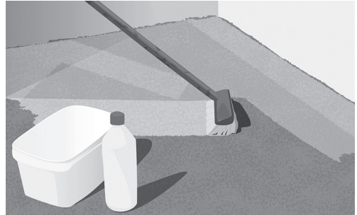
Fig. 3. Clean and prime the floor
