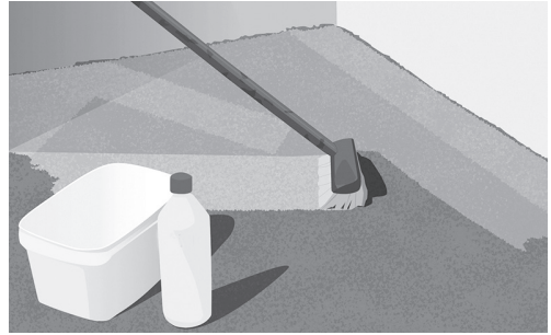
Fig. 4. Clean and prime the floor
